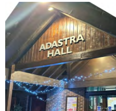
Refurbishment and signage.
