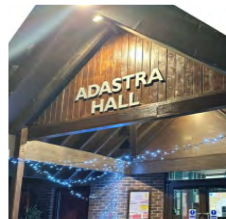
Refurbishment and signage.
